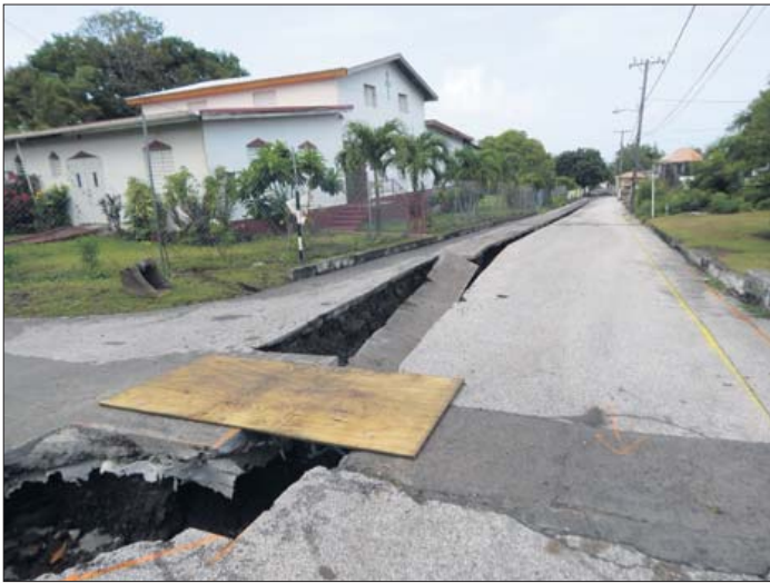
The caved-in trench on Queen Beatrix Street.
